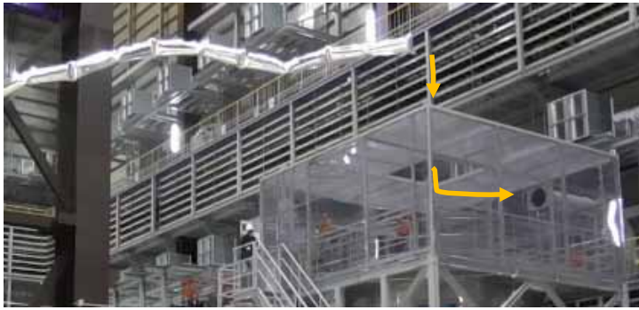
Negotiating to the roof window to approach the pipe
